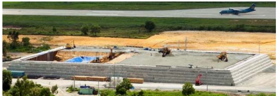
Complete containment structure, 55 percent filled (Photo: Tetra Tech)
