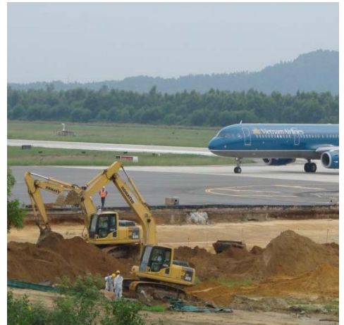
Excavating soil north of the Danang Airport runway (Photo: Tetra Tech)
